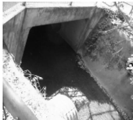
The new culvert is wider and taller than the existing culvert (7 feet by 16 feet). The road will be raised by 0.63 feet where it crosses the culvert. The road will be reconstructed for 75 feet on either side of the culvert to match the new grade. This project is expected to take about six weeks.
