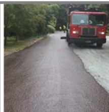
**Slurry Seal**– 62 street segments slurry sealed (1,530,000 SF
