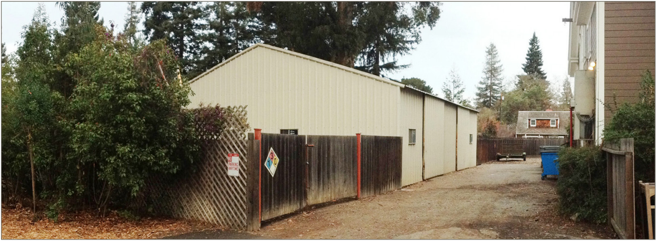
Drive between Carriage House and Corp Yard
