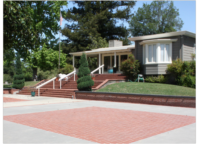
6. Brick Patio at Main House
