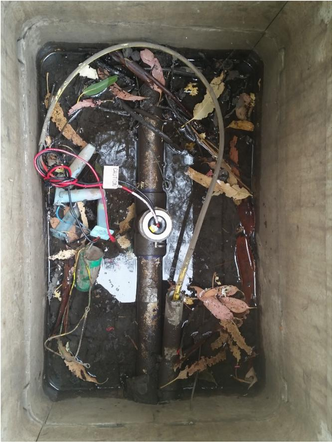
LEFT - New flow sensor installed in system adjacent to new well.
